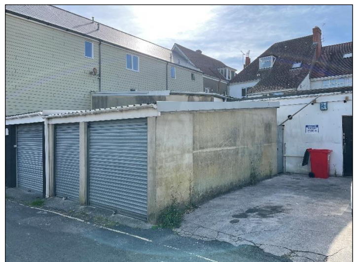
Rear entrance to Store - (Middle roller shutter door)
