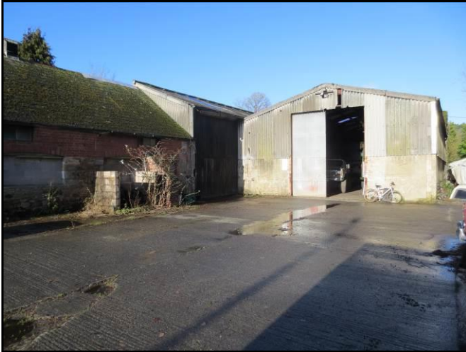
Building No 1 – To be removed and replaced.
