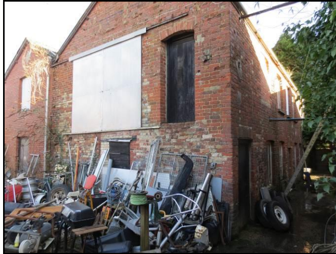
Openings in the side elevation to Building No 3
