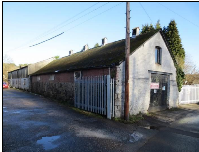
Building No2 – To be retained and converted
