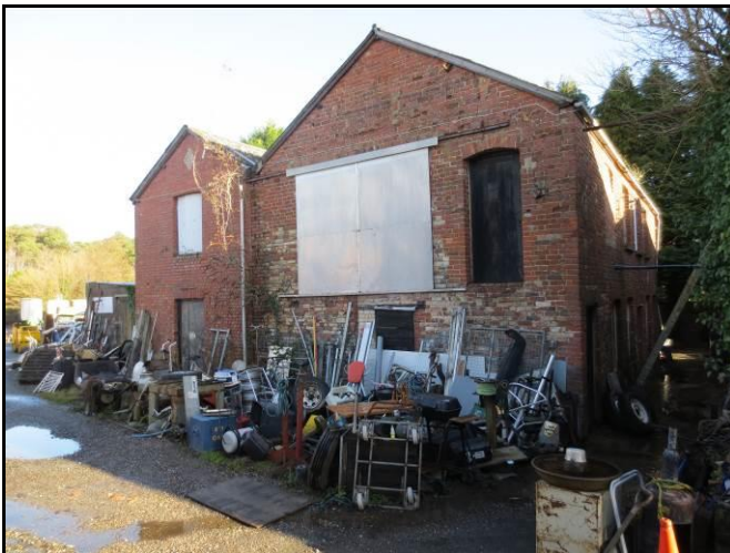
Building No 3 – To be retained and converted
